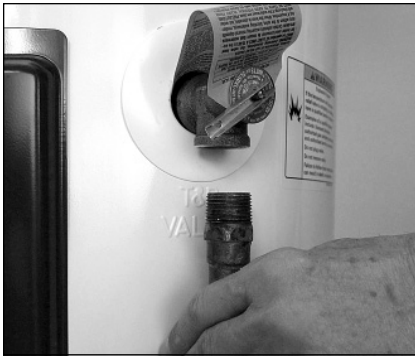
Figure 11 - Removing the T&P Relief Valve discharge pipe.
