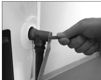
Figure 41 - T&P Relief Valve
