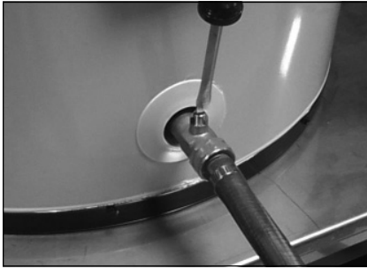
Figure 10 - Draining the old water heater.
